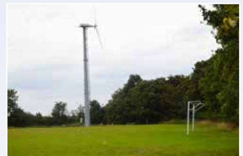
F Green energy improvements to Community Buildings such as a wind turbine at Blackbourne
